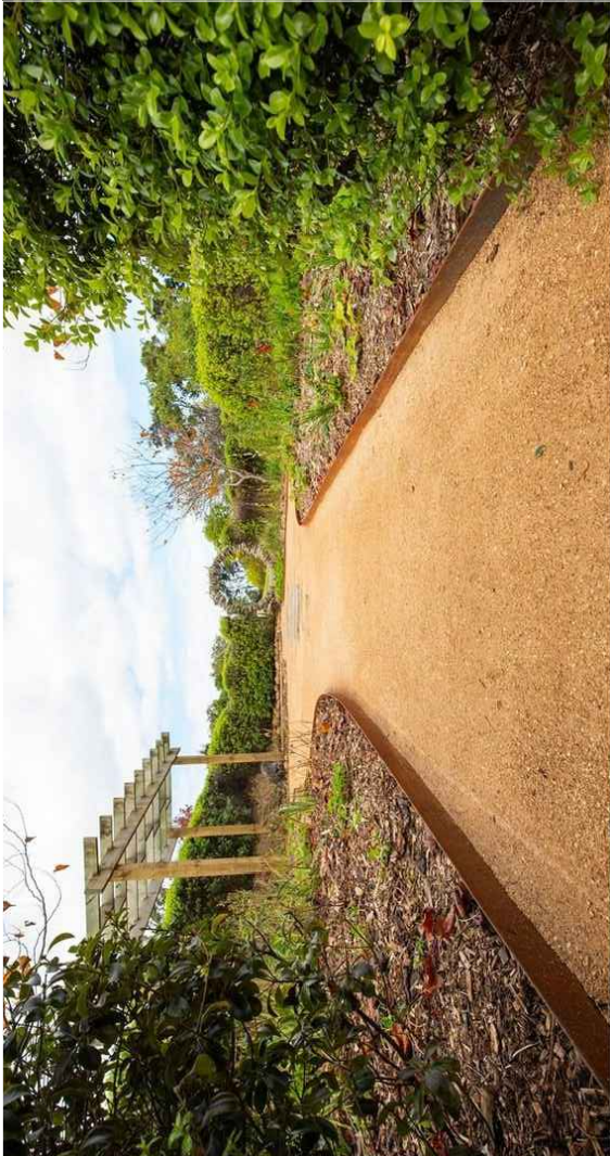
DG TO BE 3" THICK ORGANIC LOCK- GOLD, AVAILABLE AT GAIL MATERIALS. METAL EDGING TO BE GALVANIZED STEEL, AVAILABLE AT VODALAND.
